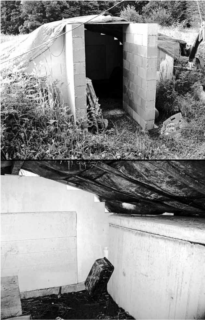
Entrance and interior of a root cellar built between two concrete water tanks made from pre-cast septic vaults. (Design by Darren and Espri Bender-Beauregard) [Credit: Keith Johnson]
