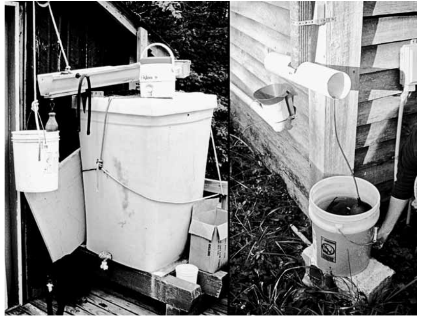
Pulley-and-pivot systems are one way to divert the first few gallons of dirty roofwater flushed by rain before directing runoff to storage. [Credit: Peter Bane]
