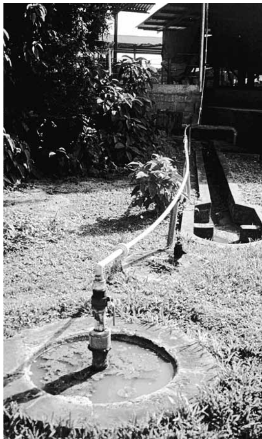
The above-ground portion of a digester that turns hog manure into methane and fertilizer.
