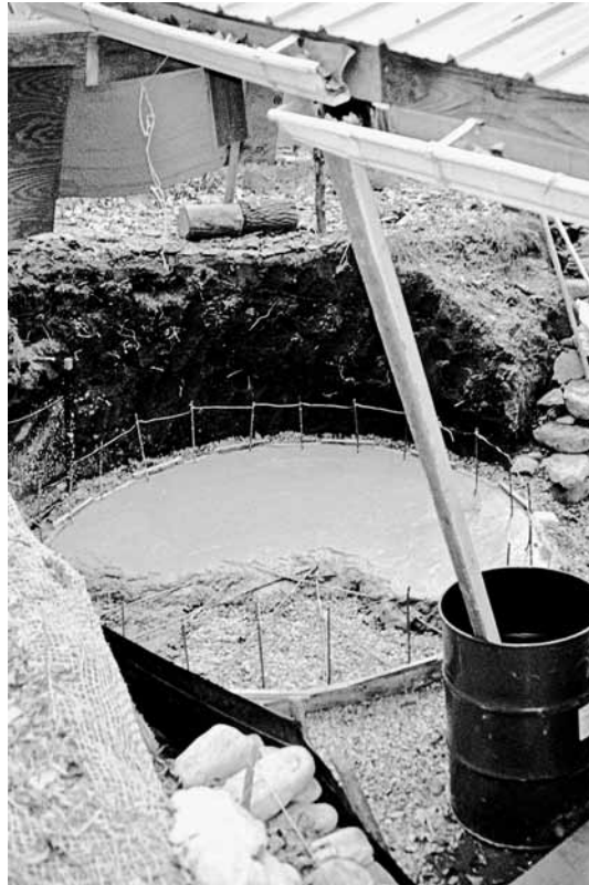
A 1,600-gallon ferrocement tank as its slab is being poured. A “spider” of rebar reinforces the slab and sticks up to form the lower reinforcement of the walls. All work on this small tank was done by hand, including concrete and mortar mixing.
