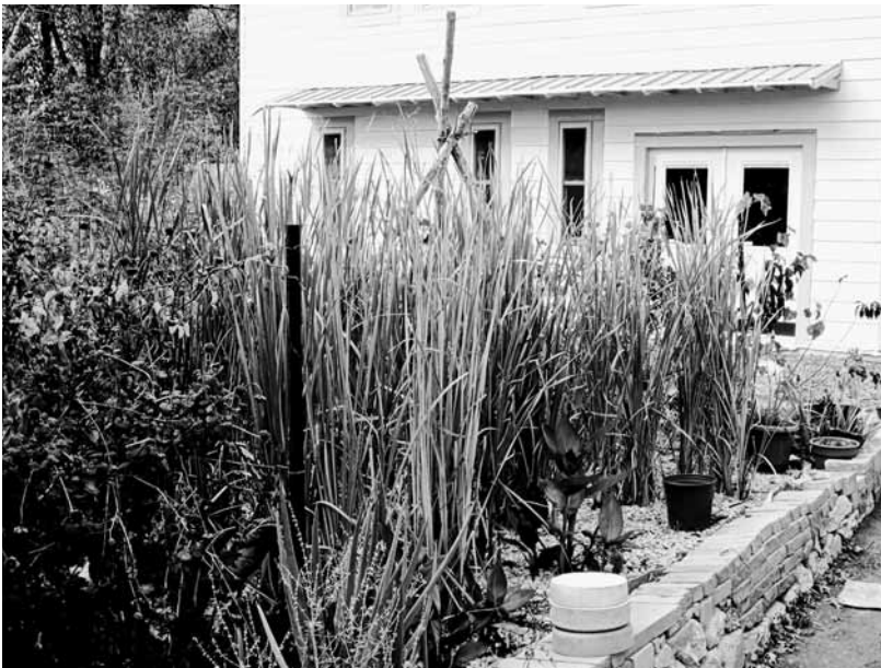
This wetland cell is populated by cattails and cannas. They grow out of the gravel medium with their roots in the subsurface wastewater. [Credit: Creighton Hofeditz]
