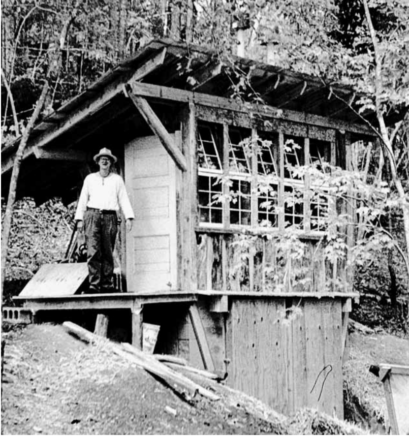
This free-standing mouldering toilet has two chambers built into a hillside. The south-facing glass front assists venting through the solar chimney.
