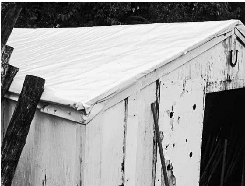
This ramshackle shed was given several years of new life by the addition of a $38 billboard tarp over a failing roof. [Credit: Creighton Hofeditz]
